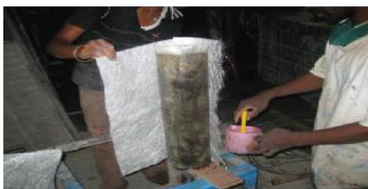
Figure 4. Wrapping under progress
