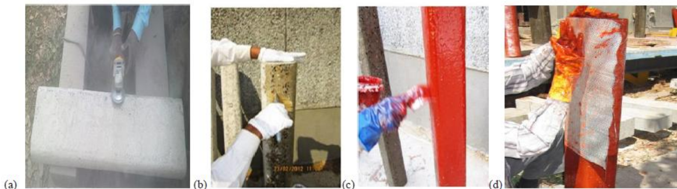
Fig. 4 (a) Grinding of RC column, (b) Application of Primer, (c) Application of saturant and (d) Application of GFRP sheet
